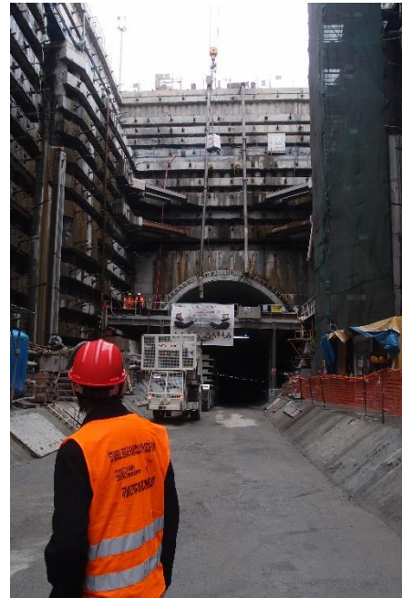
An undersea tunnel under construction
