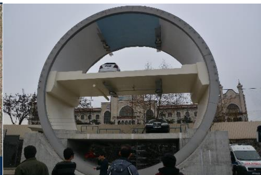
Cross section of tunnel
