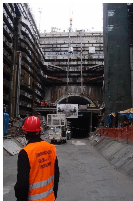
An undersea tunnel under construction
